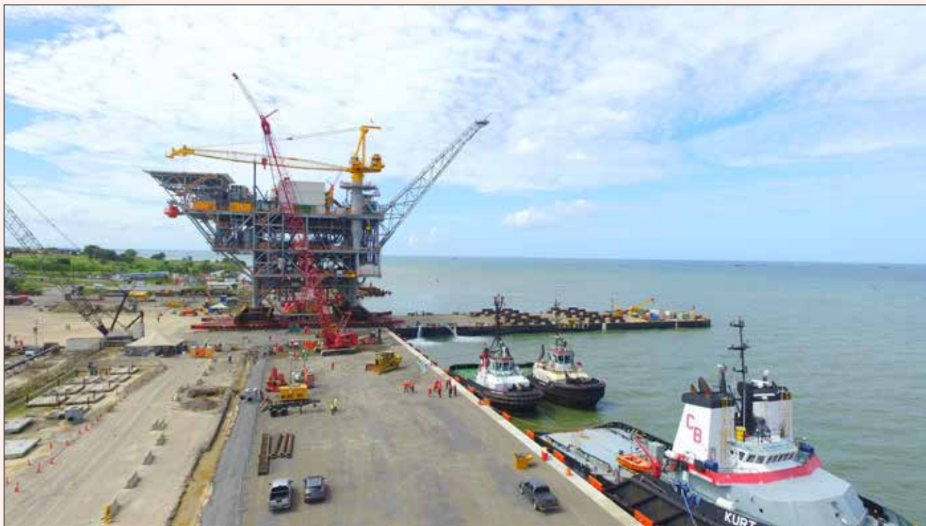
Juniper Platform is successfully loaded out from Berth 2, Port of Brighton
