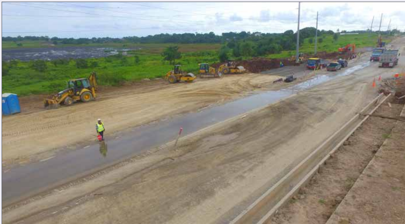
In Progress: Reconstruction of LABIDCO's corridor and pipeline ROW
