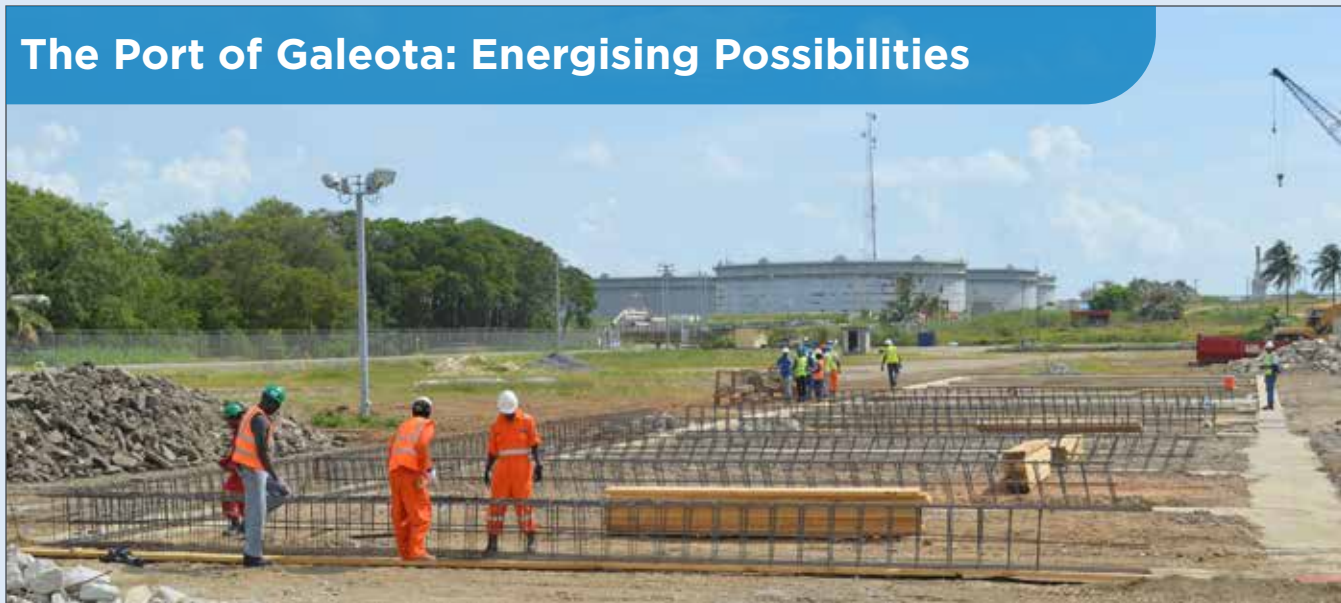
Foundation works ongoing for Port of Galeota's Warehouse Building
