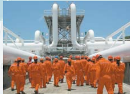
Participants in the Natural Gas Tertiary Level Workshop tour the Beachfield Slug Catcher Facility
