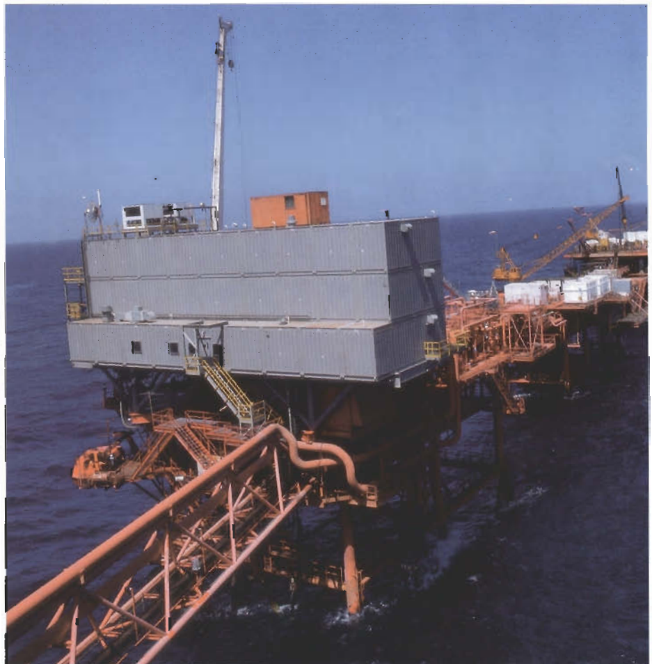
BP installation off the south-east coast of Trinidad.
