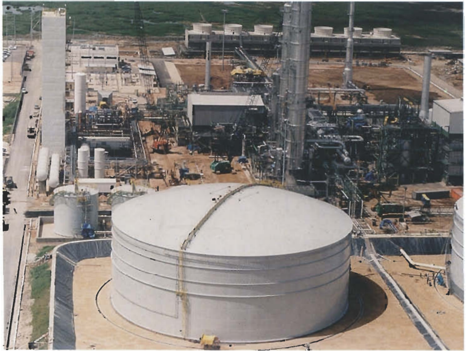
Titan Methanol Company, Pt. Lisas Industrial Estate.
