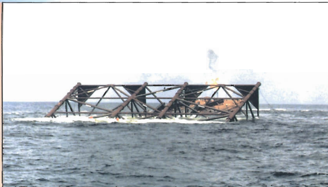
Jacket for platforms being off-loaded by barge - south-east coast of Trinidad.
