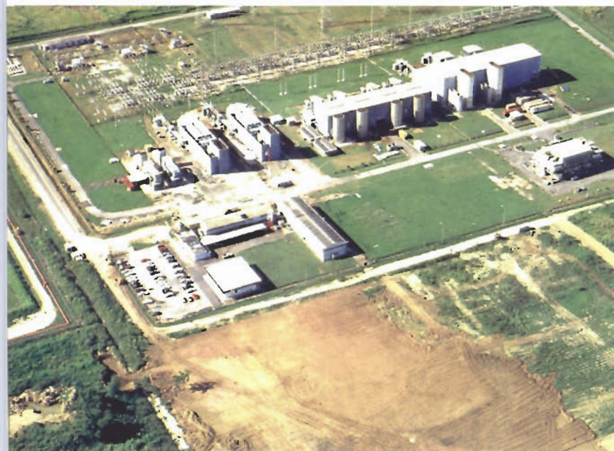
Aerial View - Power Generation plant at Point Lisas.
