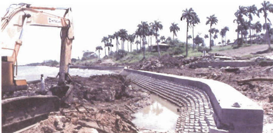
Shore Protection works at new industrial site at La Brea
