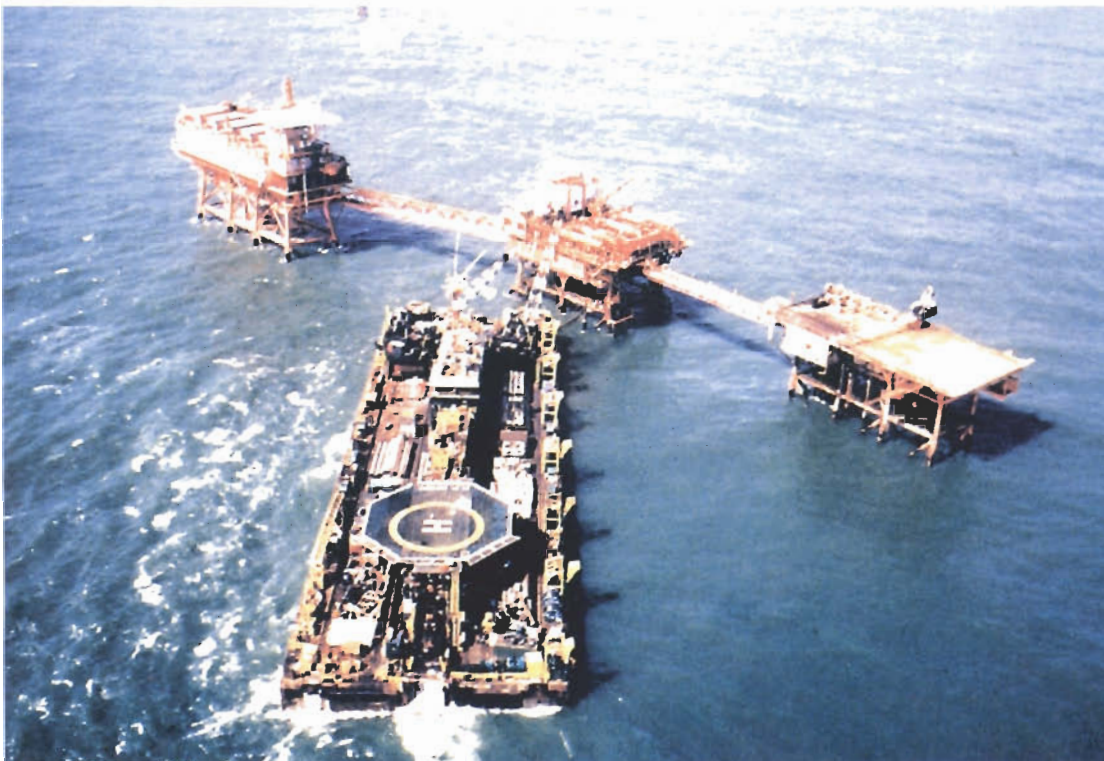
Solar Compressors were brought by barge
