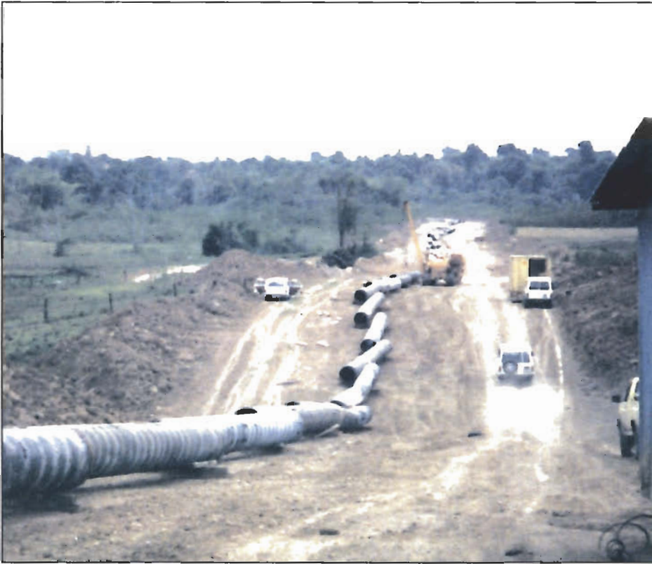
Construction work on the 30" \phi cross country pipeline in 1983.
