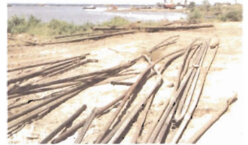
Removal of old infrastructure from industrial site
