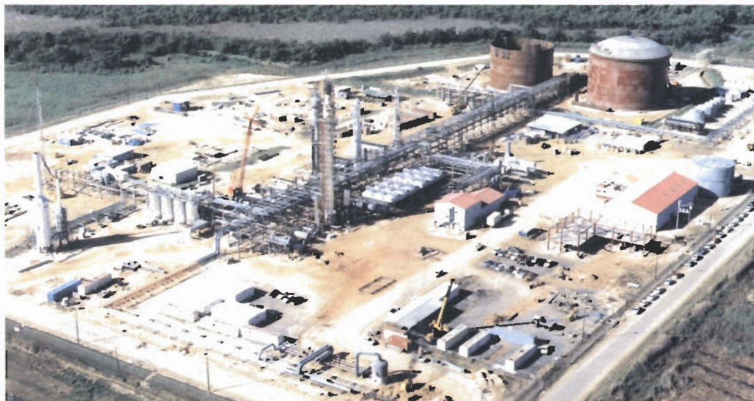
Phoenix Park Gas Processors Limited under construction
