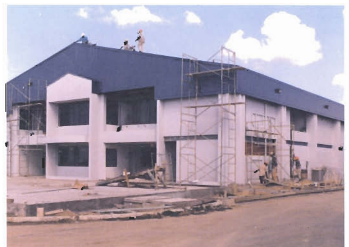
1994 - Field Office in construction phase
